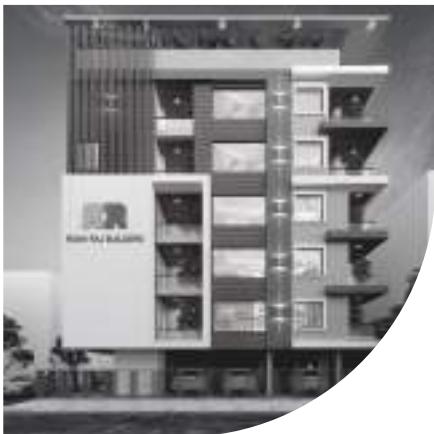
BUNGLOW 4 A-25, Nemi Nagar, Vaishali Nagar, Jaipur
