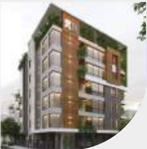
BUNGLOW 5 Behind Gandhi Path, Queens Road, Vaishali Nagar, Jaipur
