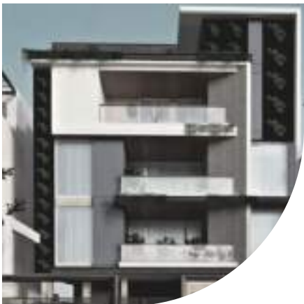
BUNGLOW 4 A-24, Nemi Nagar, Vaishali Nagar, Jaipur
