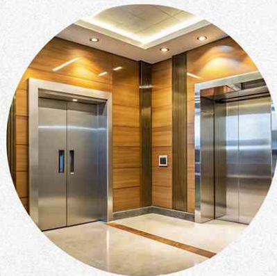
State-of-art Vertical Transportation: Two High Speed Lifts.
