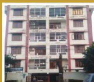
DEEP SHREE APARTMENT 122, Shakti Nagar
