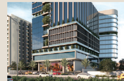
CHORDIA'S THE KAIRO SHOWROOMS/OFFICE SPACES AT MAIN SODALA
