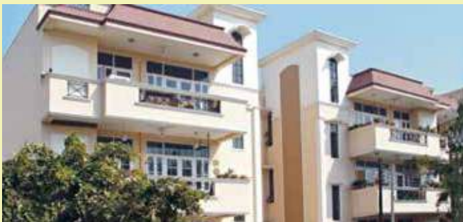
CLASSIC PERSONAL FLOOR, GURGAON
